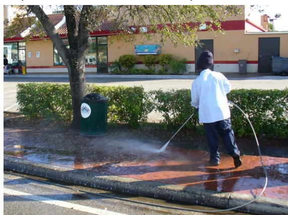
Pressure cleaning of sidewalks on NE 6th Ave
