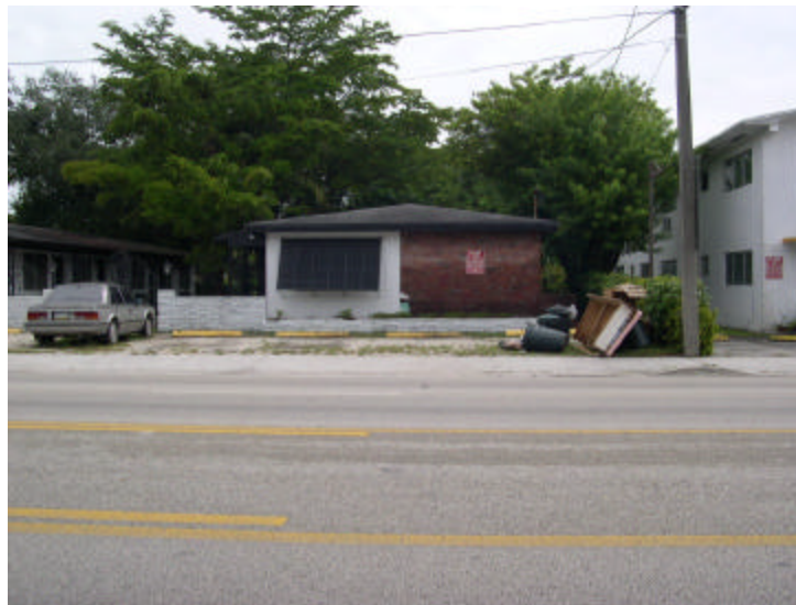
Junk and trash present on site
