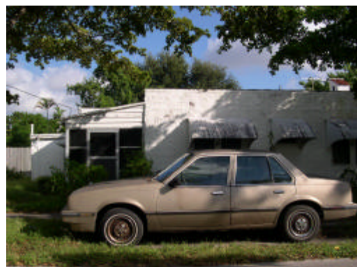
Broken awning; rotted structure
