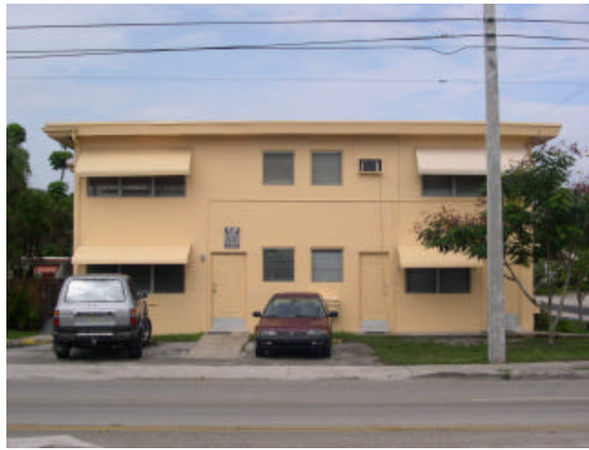
Backing into traffic; inadequate open space (16NE6thAve)
