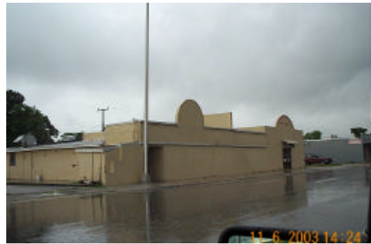
Functionally obsolete commercial buildings
