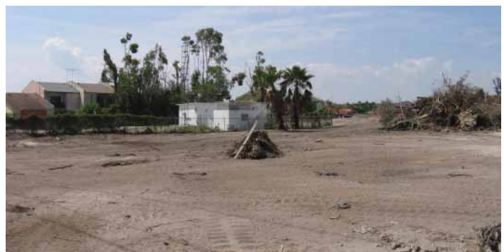
Before and After: Clearing the Ruck's Park site for development.
